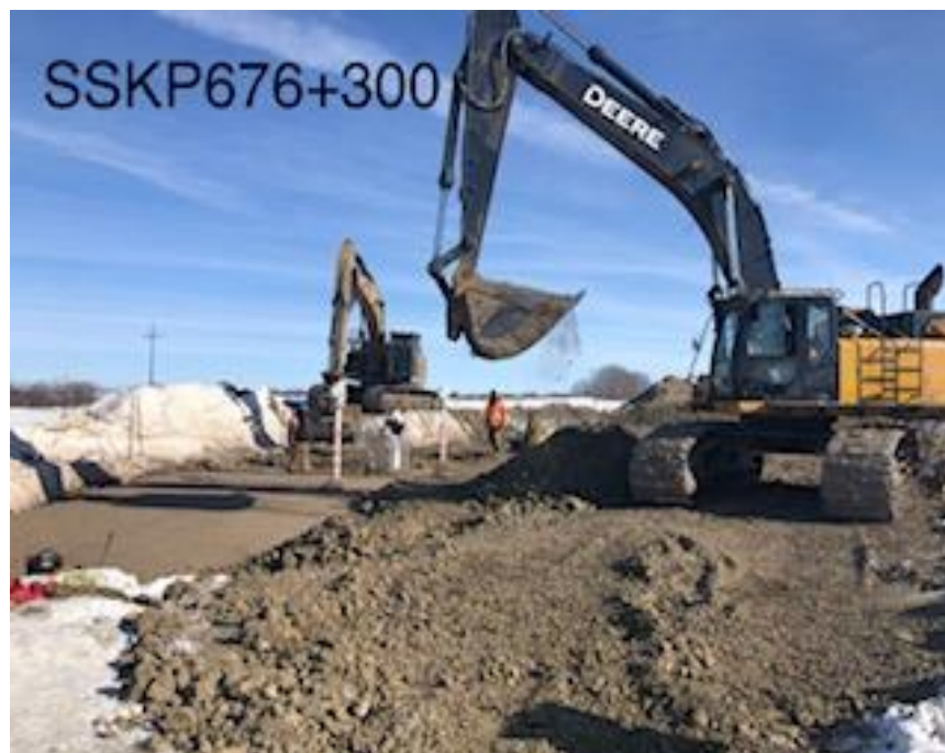
Sand compaction completed, backfilling MLBV 17 valve station with subsoil from trench area - Final lift reached!
