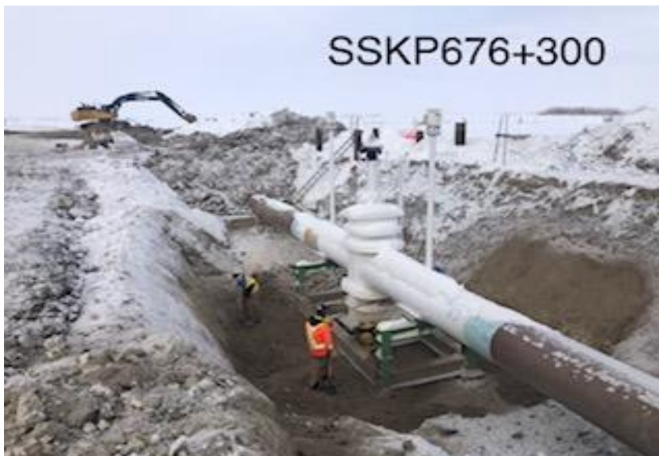
Compaction started at MLBV17 – sand fill worker breaking down hard clay with hand shovel before use of compaction plates.
