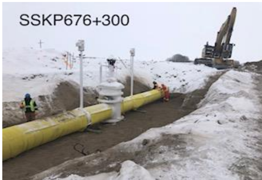
Workers applied rock shield - rock shield is a plastic mesh used as pipe guard to protect pipeline from rocks when backfilled. Rocks can easily damage the pipes protective coatings and the rock shield mesh helps to cushion any impact during the backfilling.
