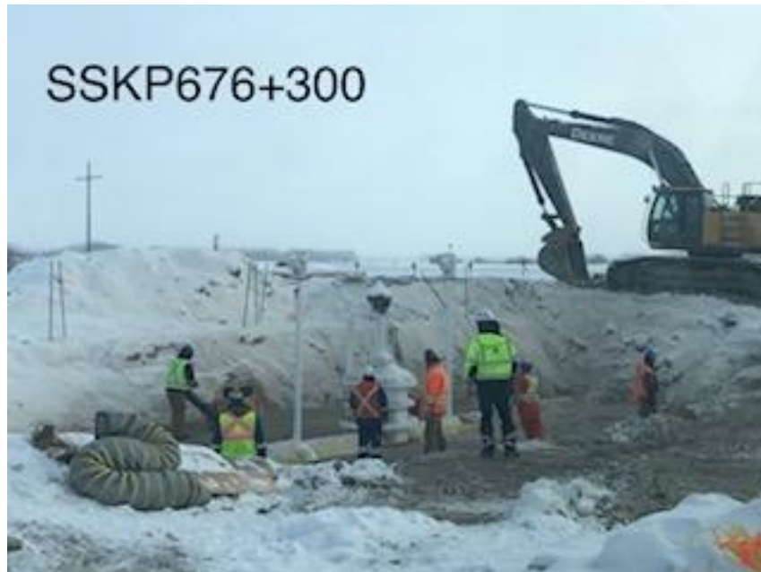
Pinter & Associates LTD employee conducting compaction test testing 5 areas in the pad area after each lift
