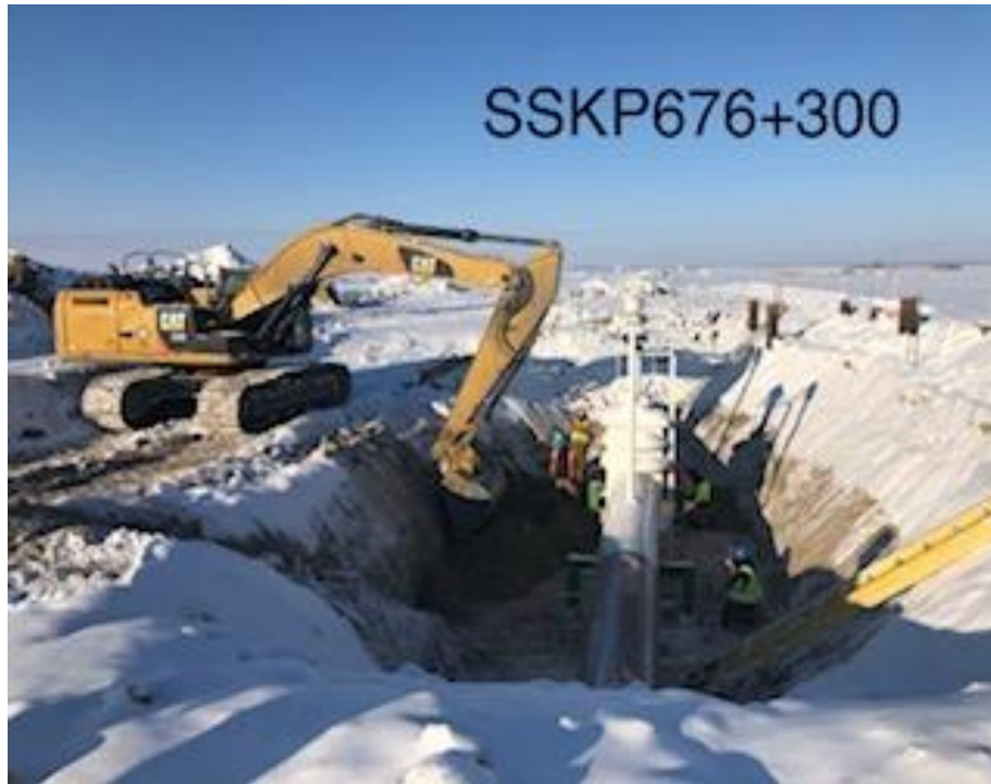
Sand fill being shaded in by bucket – spotter inside trench area used whistle to alert other workers during the backfill process. (Safety feature)
